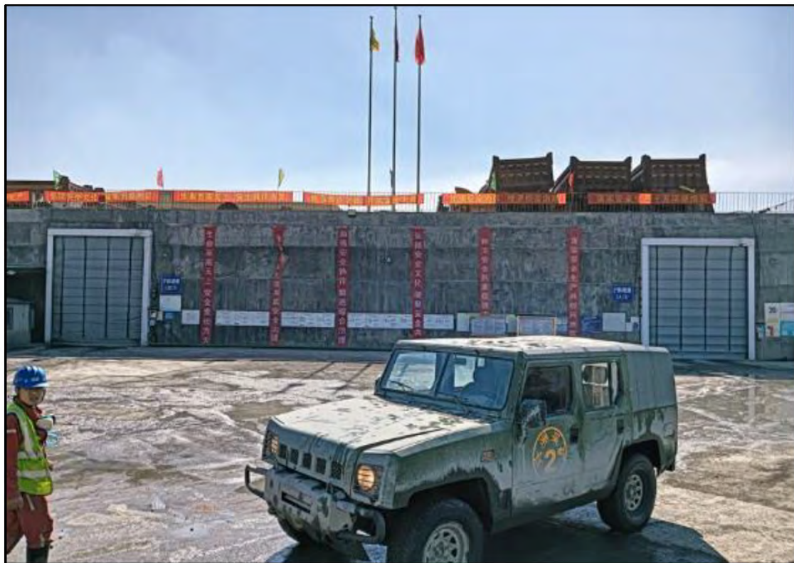
Figure 15-3 Portals to underground workings.
