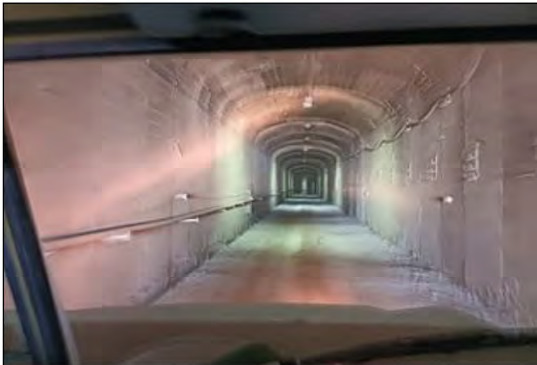
Figure 15-5 Access decline to underground workings.
