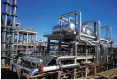
We use the “two-stage CLAUS + selective hydrogenation + selective oxidation” process, with a total sulfur recovery rate above 99%.
