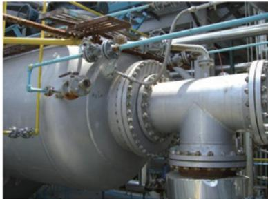
Burner used in SRUs is responsible to mix fuel gas, acidic gas and combustion air into a definite form and product combustion reaction by spraying the mixture into fire channels and furnaces. Efficient burners can improve the conversion rate of elemental sulphur in thermal reactors, eliminate the influence on downstream equipment from heavy hydrocarbon of ammonium salt or other impurities and ensure efficiency and reliable operation of SRU equipment.
