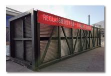
The product's core is made of glass tube and the shell is made of metal with anti-corrosion coating. It is mostly used in flue gas de-whitening projects. Compared with modified polymer material, glass tube heat exchanger has better heat and corrosion resistance.
