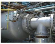
Sulphur condenser forms the shell and tube boiler of a special type of heat exchanger. The main function is to cool down sulphur generated in the upstream reaction section of heat exchanger systems.
