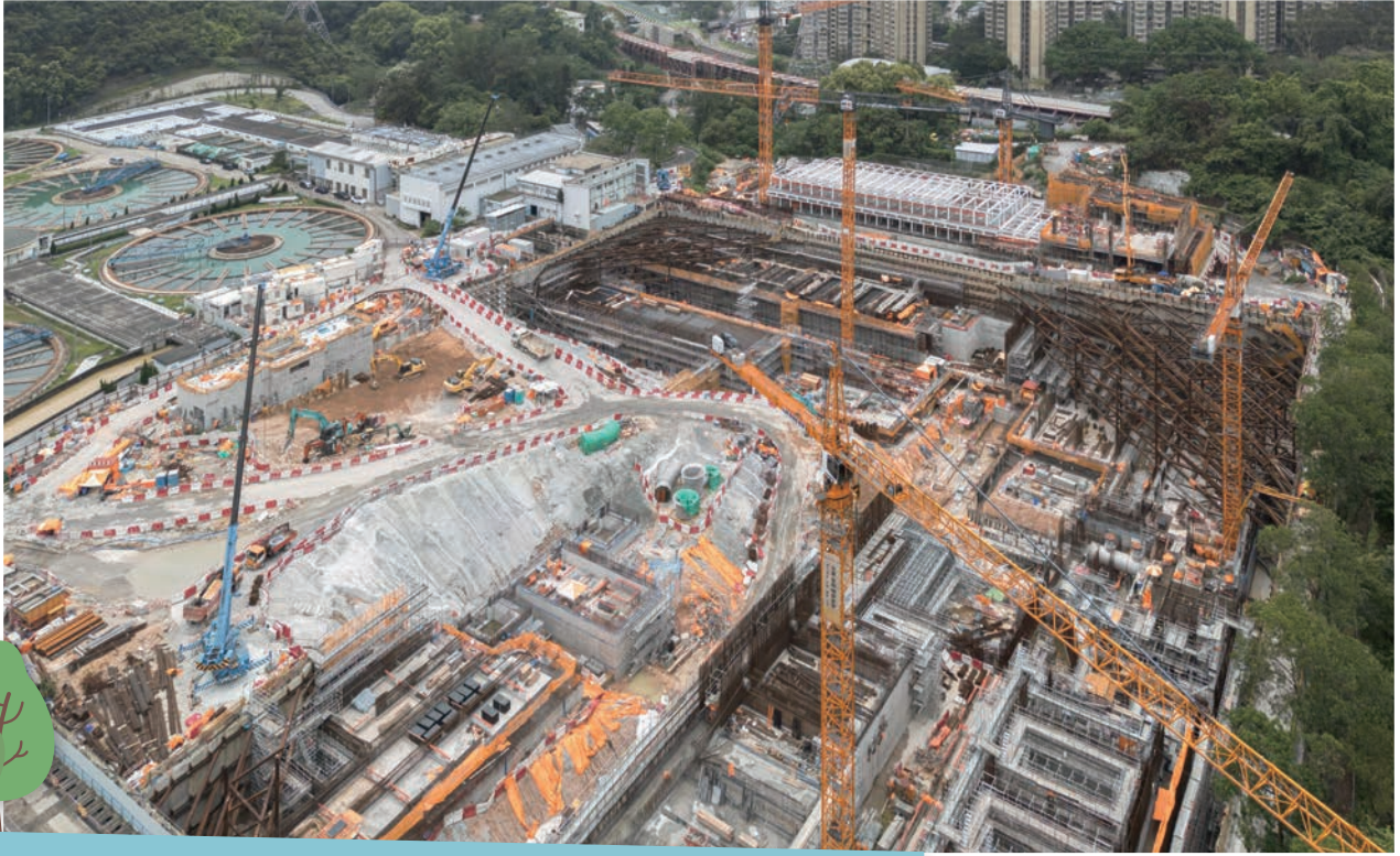
In-situ Re-provisioning of Sha Tin Water Treatment Works (South Works) — Water Treatment Works and Ancillary Facilities 沙田濾水廠原地重置工程(南廠) — 濾水廠及附屬設施
