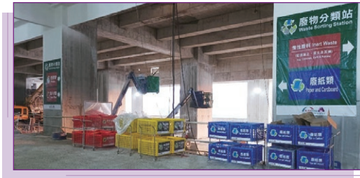
Set up waste sorting stations to improve cleanliness and tidiness of sites 設立廢物分類站，以改善地盤的整潔度
