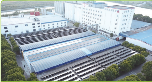
◇ The solar PV modules installed in the flour plant in Jintan 於金壇麵粉廠所安裝的太陽光伏組件
