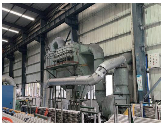
Production plants equipped with dust collectors with filter bags 生產廠房中設有布袋除塵器
