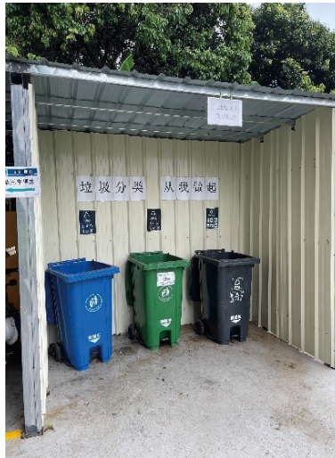
Waste separation facilities for recyclable, non-recyclable and hazardous wastes in the factory area 在廠房園區已設置可回收垃圾、不可回收垃圾及有害垃圾廢物分類設施
