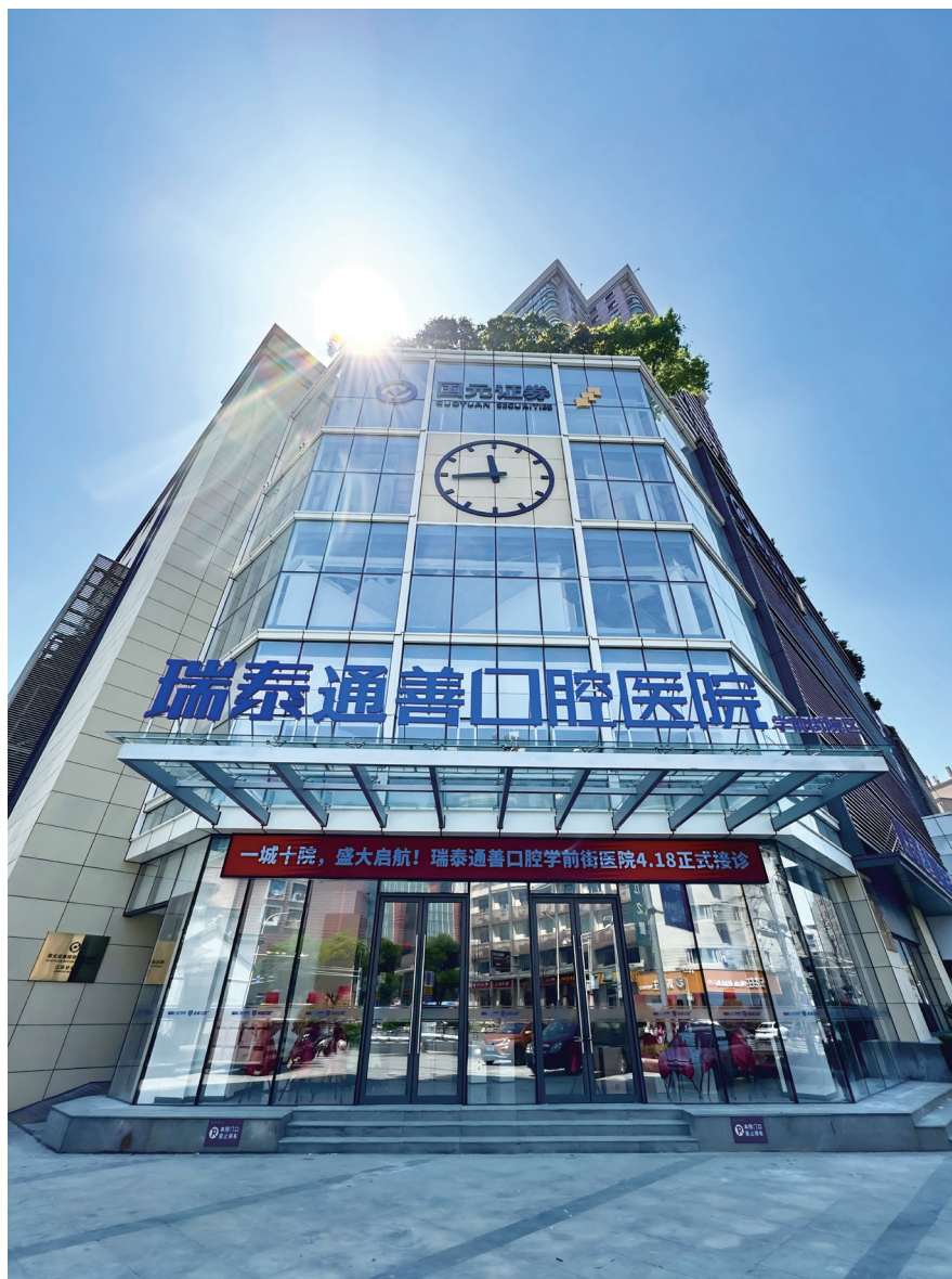
Rytime Tongshan Xueqianjie Hospital 瑞泰通善口腔學前街醫院
