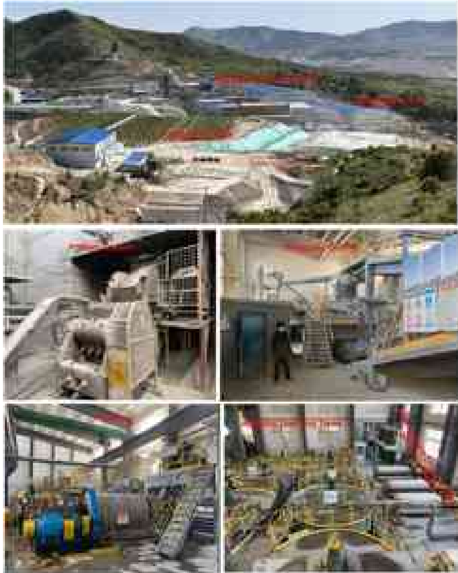
Figure 11-2: Site Photos of #1 Jilong Plant
