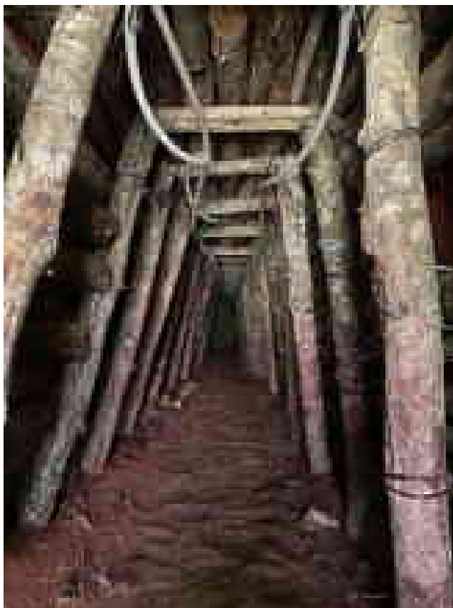
Figure 12-7: Main PLS Collection Tunnel in Construction
