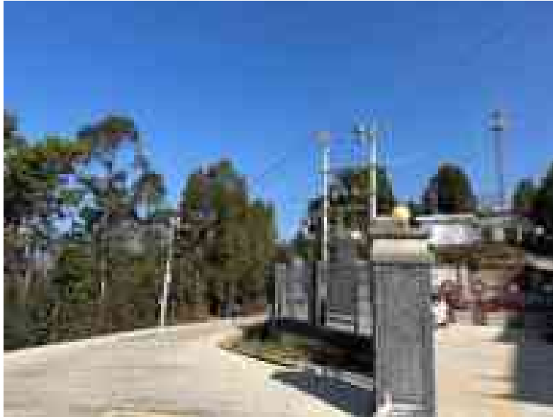
Figure 12-1: Power Station of Liantiexiang
