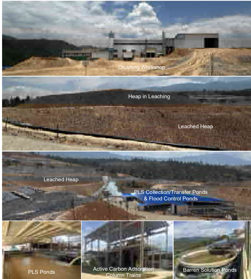
Figure 11-15: Main Facility Photos of Xidengping Heap Leach Plant
