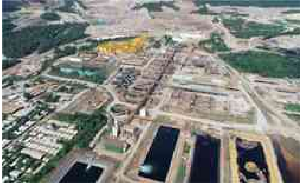
Figure 13-1: Sepon Gold Plant and Copper Plant Complex
