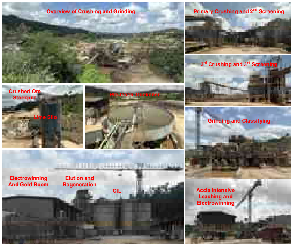
Figure 13-2: Photo of Wassa Processing Plant
