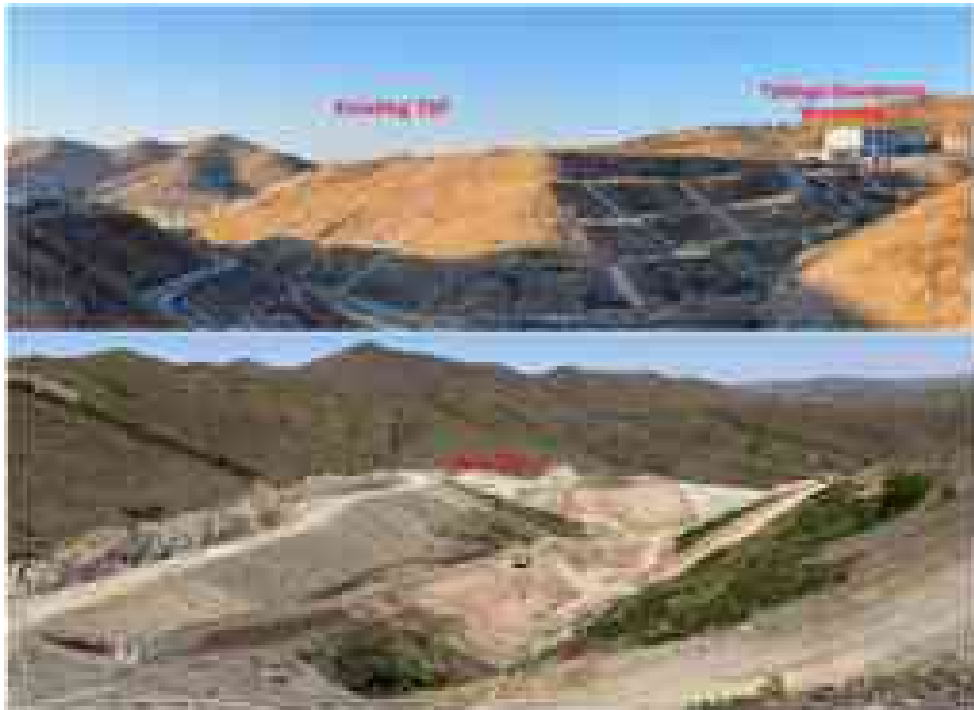
Figure 11-4: TSF of Jilong Project
