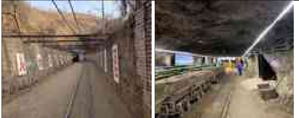
Figure 10-6: Photos of Main Adit Portal and Shaft Station on Level 5
