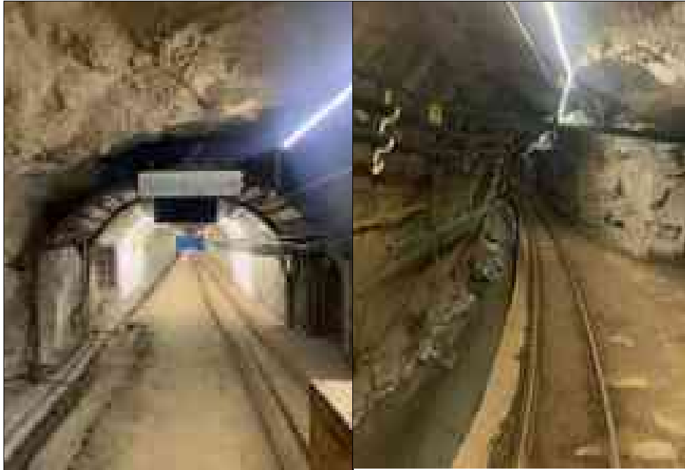
Figure 10-20: Photos of Access of Adit and Drift on Level 3 at Dongfeng Mine
