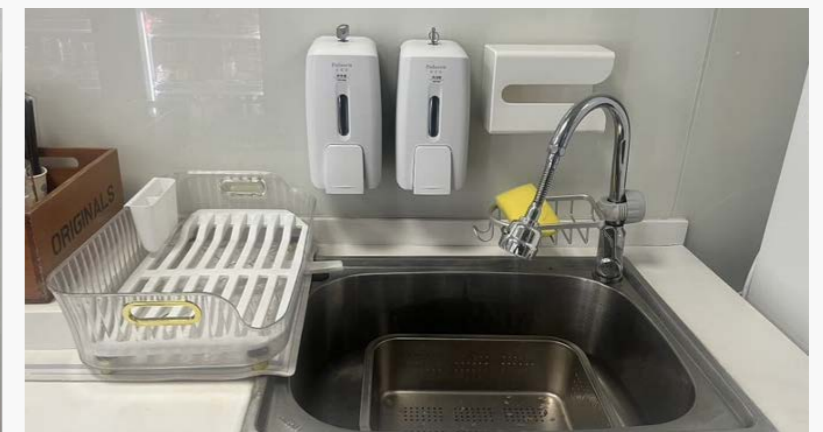
Installed Water Savers on Faucets
