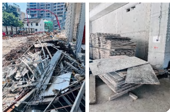
On-site sorting location for construction waste (steel, gypsum board and timber) at Westlake 66
