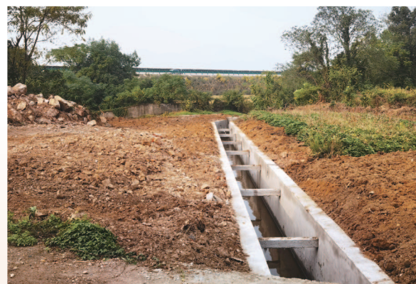
Repairing concrete ditch in Pingding Village, Yanqiao Town
