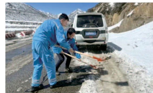
Clearing Snow on National Highway 318
