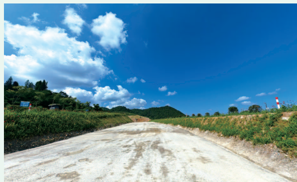
Construction of water-stabilised roads
