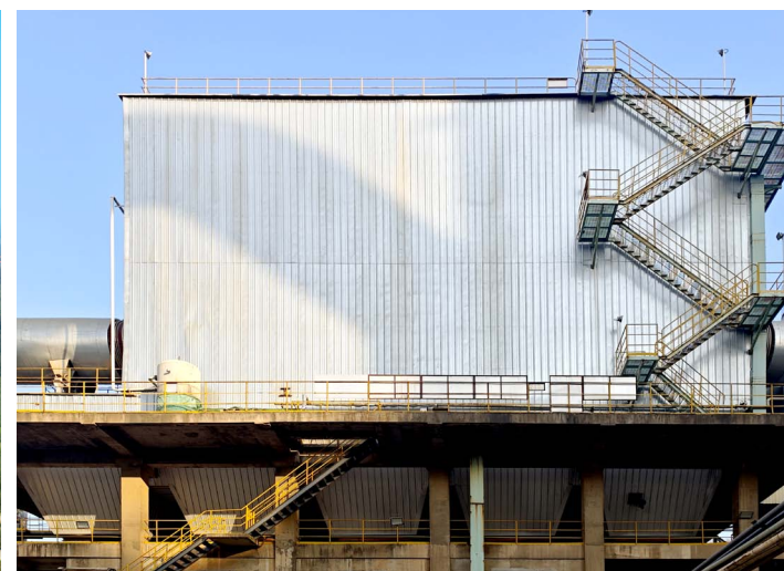
Conversion of electric dust collection to bag collection
