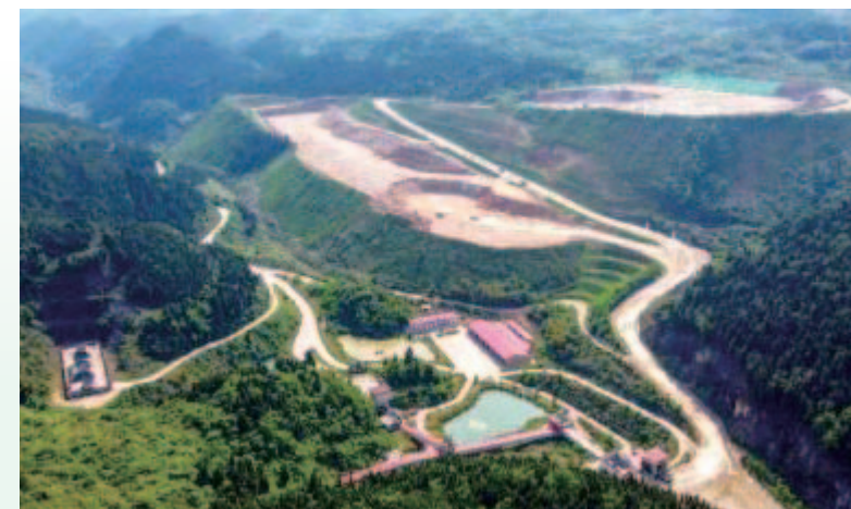
Liangping Conch Cement Mine
