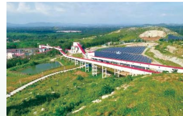
Closed crushing plant, corridor
