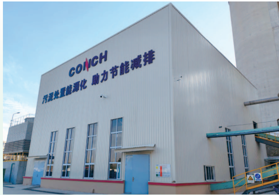
Chaohu Conch Cement Kiln Co-disposal Project
