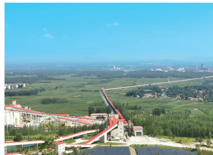
Dust control — closed crushing plant and corridor
