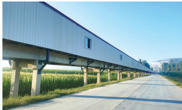
Closed conveying corridor
