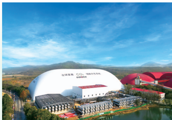
Carbon dioxide energy storage demonstration project
