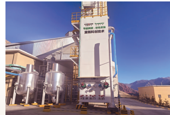
Oxygen-Enriched Combustion Transformation Project
