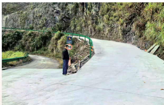
Cement hardening treatment for Fuwo Road in Wangren Town
