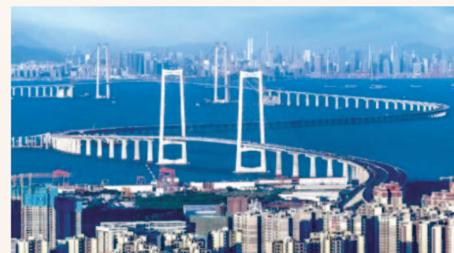
Shenzhen-Zhongshan Bridge (SZC) Railway guarantee supplied by Yingde Conch
