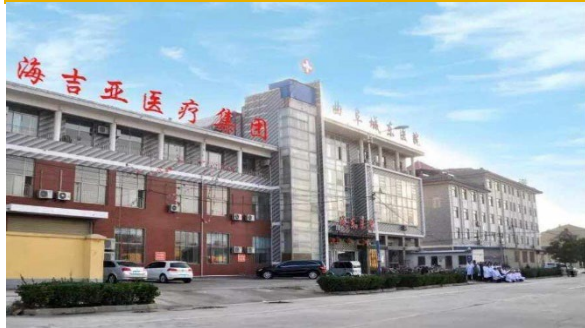
Qufu Chengdong Oncology Hospital
