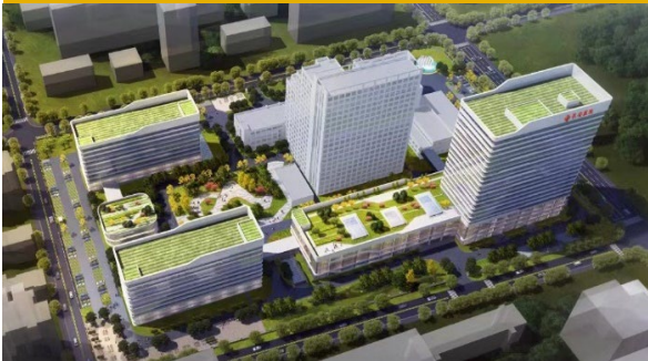
Chang'an Hospital Phase III project
