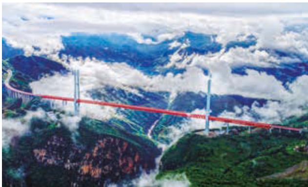
▲ The Bank's Guizhou Branch supported the construction of all projects along the Bijie-Duge Expressway
