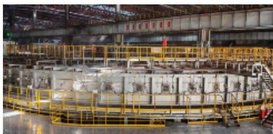
Ring furnaces after the renovation
