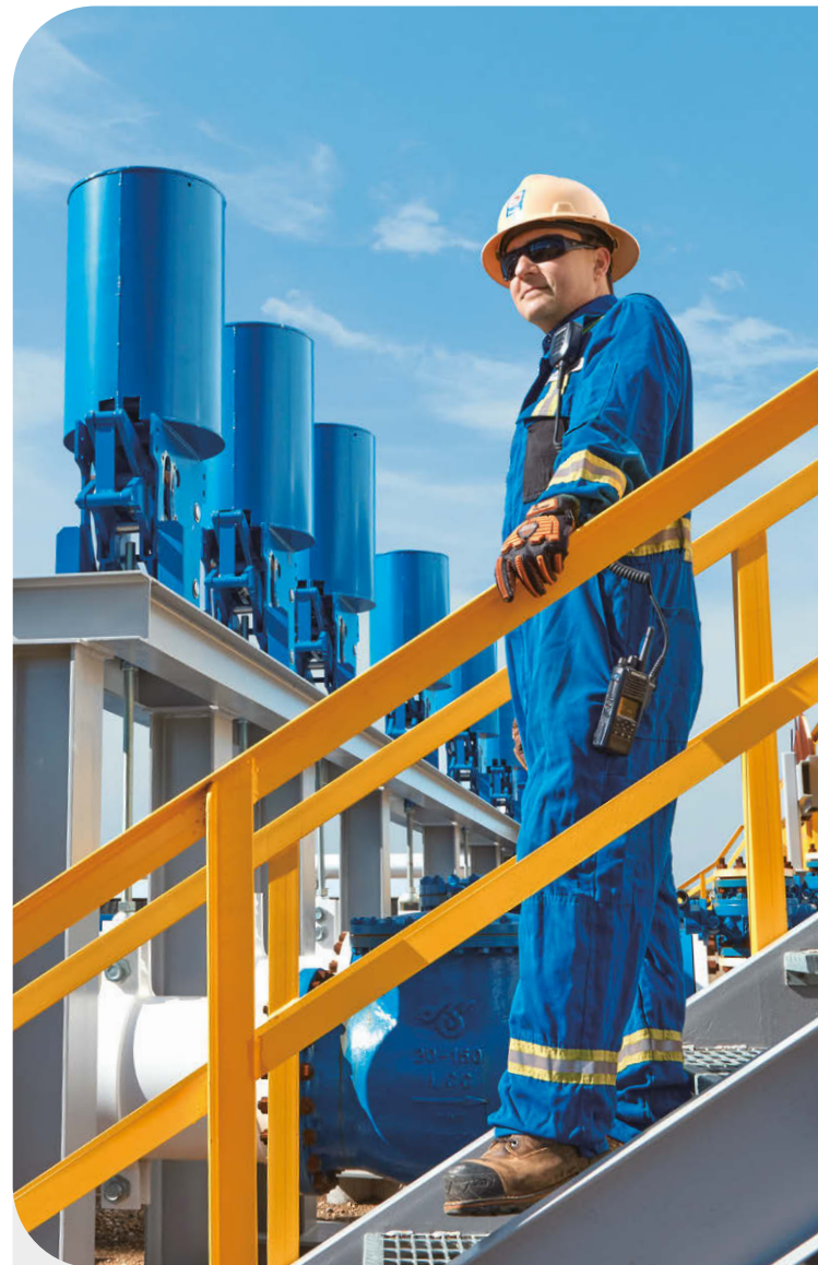
✦ An employee at Husky Midstream's oil storage terminal at Hardisty, Alberta, which has a total storage capacity of around 4.9 million barrels.
