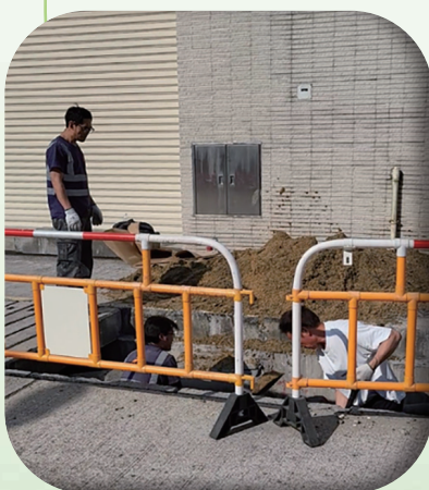
Freshwater pipelines undergoing repair works 淡水管道進行修復工程
