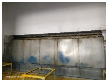
Water Curtain System for collection of spray paint exhaust
