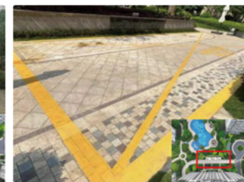
整改後 After renovation
