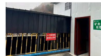
Mine Water Inflow Treatment Station of Xihe Zhongbao
