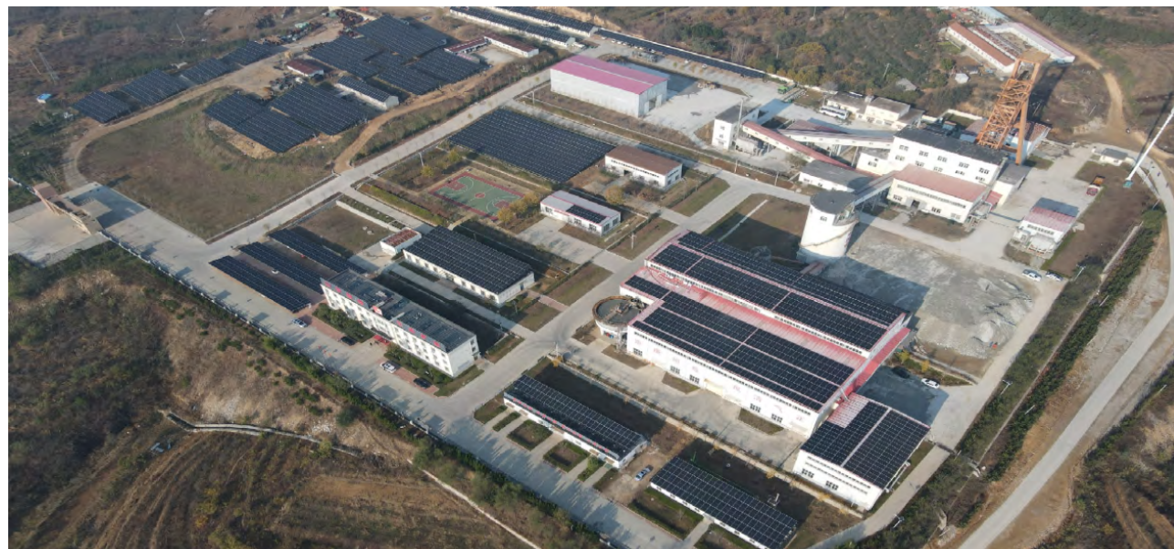
Laixi Company's Photovoltaic Power Stations Project
