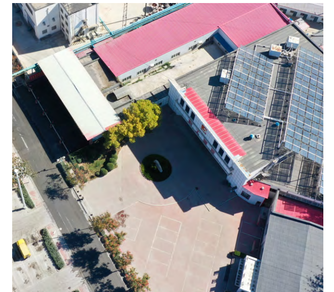
Installation of Solar Hot Water Facilities at Xincheng Gold Mine
