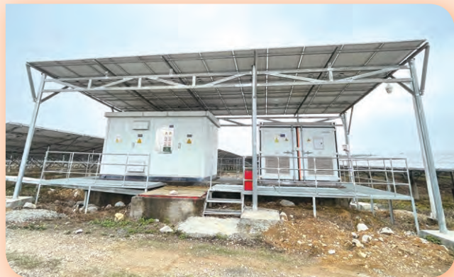
Project on the reuse of components as canopies for box transformers at Guangxi Guigang Power Plant 廣西貴港電站組件利舊箱變遮陽棚項目
