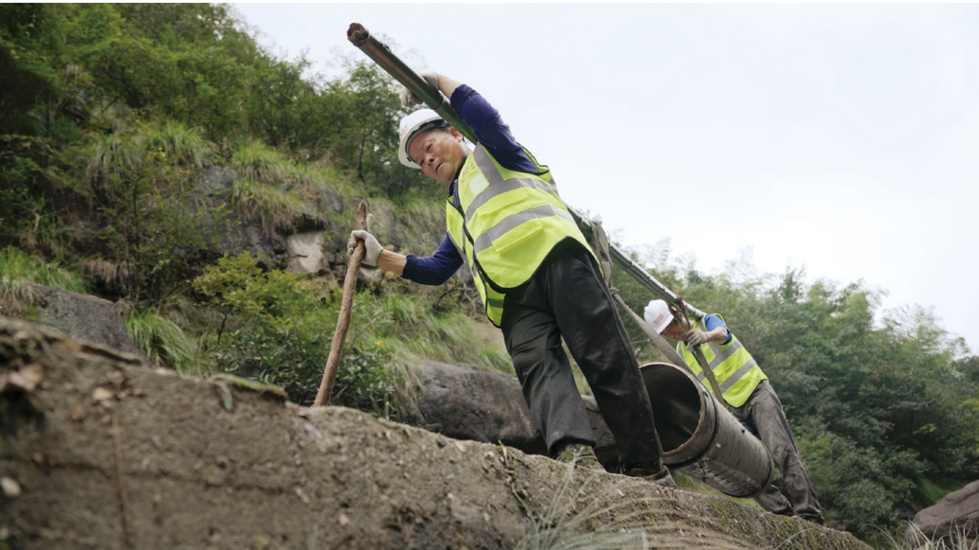
Construction of the Huangshan factory in Anhui, workers transported water pipelines by carrying them on their shoulders or by hand.
