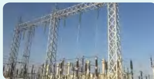
Djibouti Railway Electrification Project
