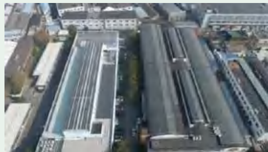
Installation of Distributed Photovoltaic Power Generation Systems on Rooftops
