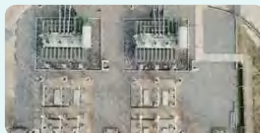
Three Transformation Stations in the First Phase of the World Bank Project in Nigeria Have Successfully Delivered Electricity
