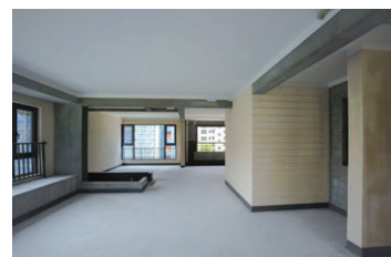
使用石膏砂漿的牆面 Walls Finished with Gypsum Plaster
