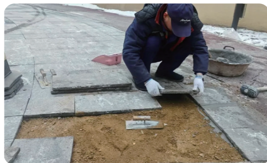
Ground Paving of Dongyuecheng North Community
