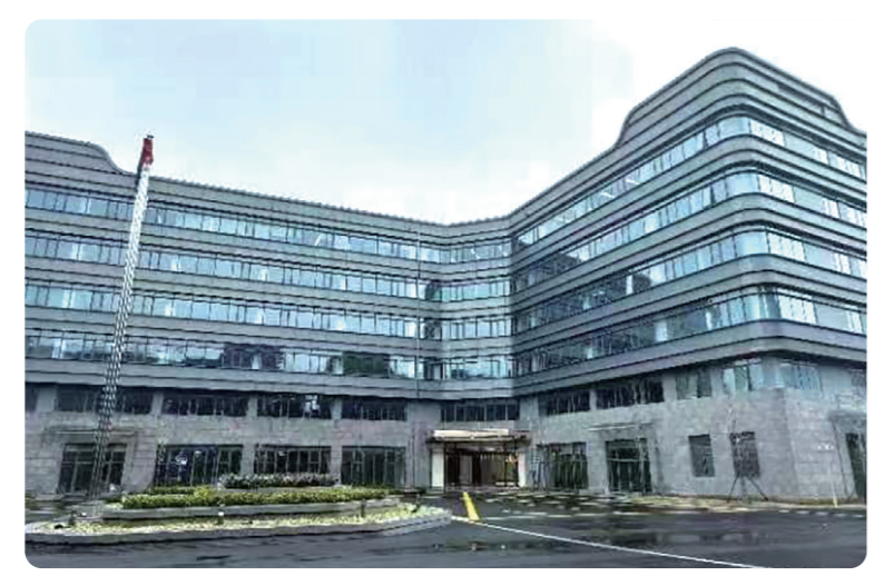
Ever Sunshine Services - Sanwang Communication Park in Songjiang District, Shanghai
