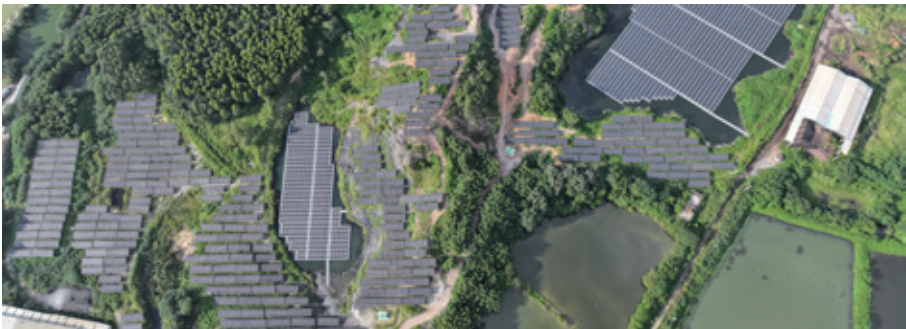
Photovoltaic Power Generation Project of Zhujiang Cement
