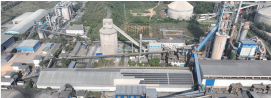
Alternative Fuel Project of Yangchun Cement
