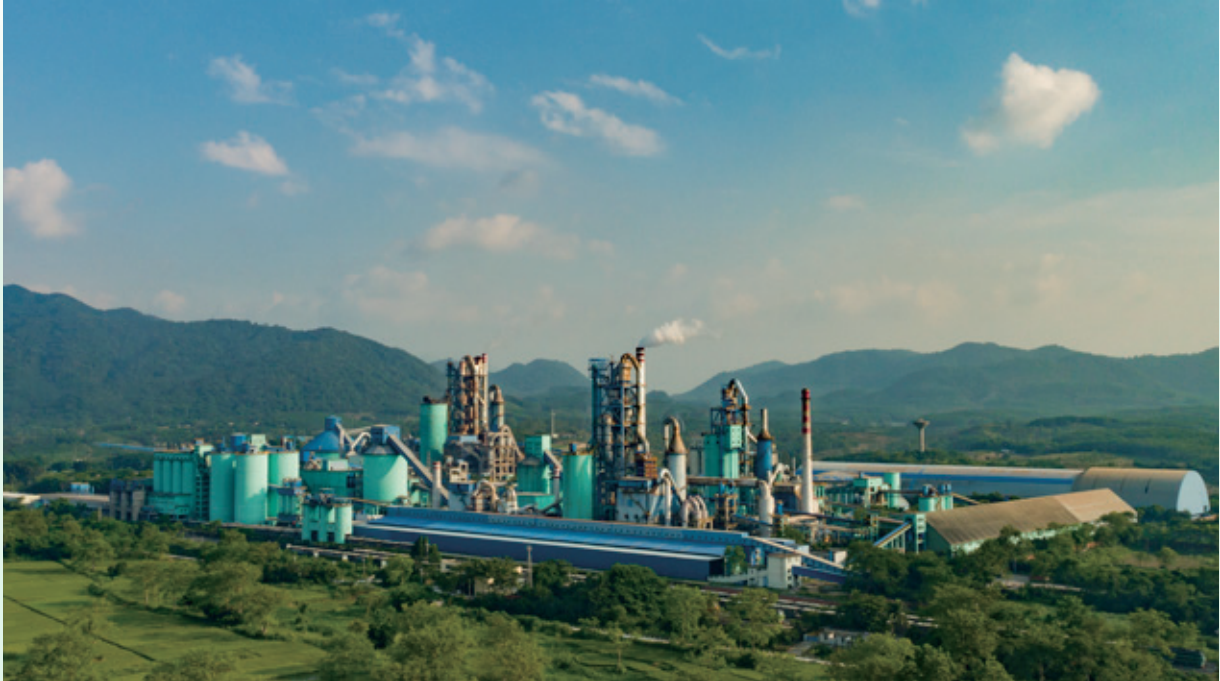
Jinjiang Cement Grinding Station at Changjiang Industry Park
