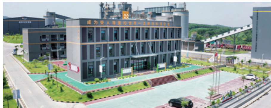
Construction waste disposal site at Changjiang Industrial Park
