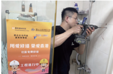
Launched the Repair and Build Hong Kong SAR community free repair initiative
