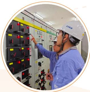
Inspection against Typhoon Yagi at Xuwen Photovoltaic Power Station
