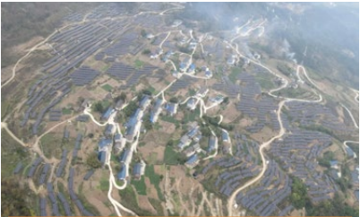
Aerial view of Jiuwanxi PV Power Station
