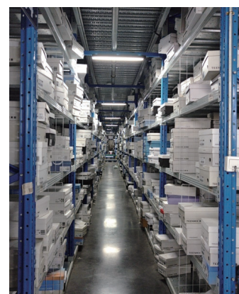
Warehouse motion sensor lighting installation
