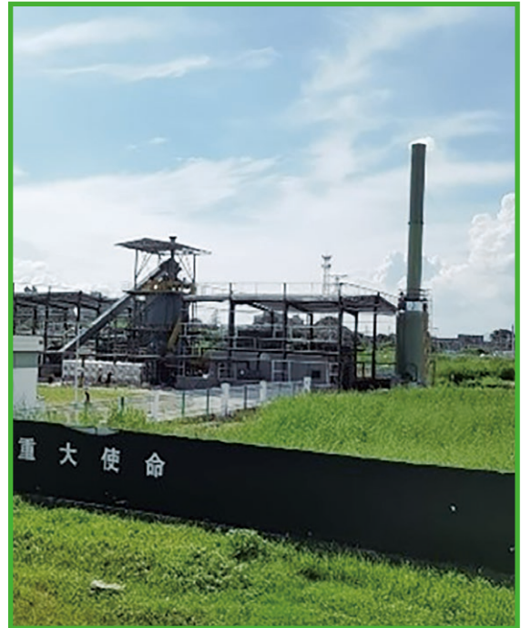
Biomass clean heating plant of Zhangzhou China Gas New Energy Technology Co., Ltd.
