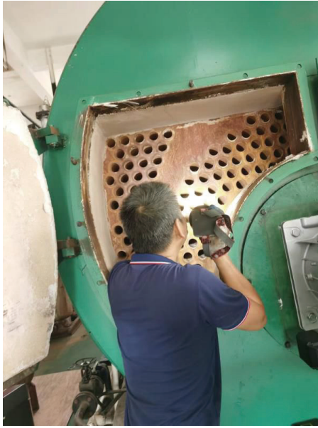
4T Boiler retrofitted with low Nitrogen Oxides burner
