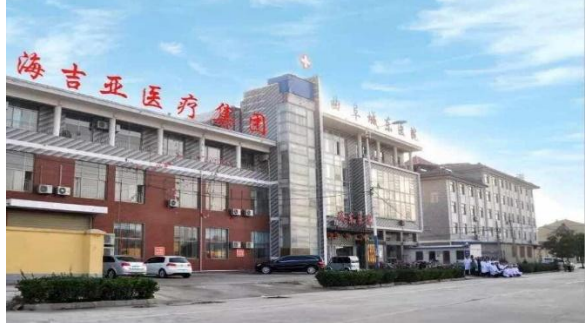
Qufu Chengdong Oncology Hospital
