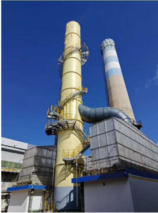
Horizontal desulphurisation of flue gas by ultrafine droplet electrolysis technology
