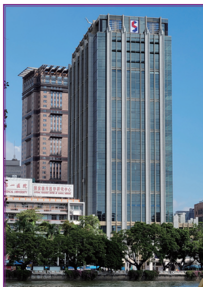
• Guangzhou Lai Fung International Center
