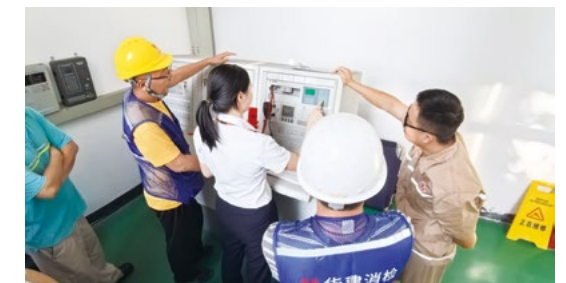
Fire automatic alarm system operation training
