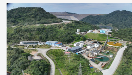
Acidic Water Treatment Plant in Dexing Copper Mine Mining Area
