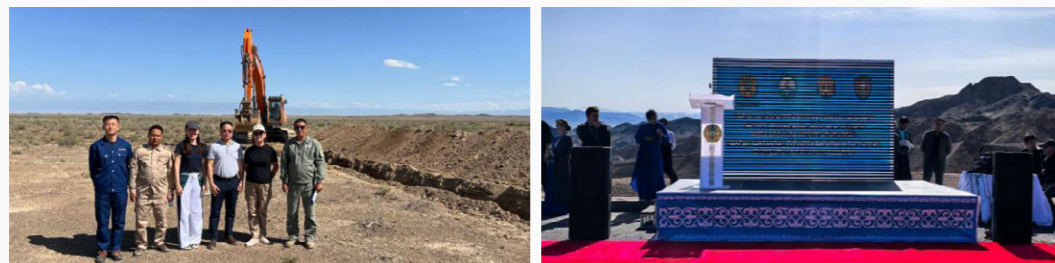
Construction and Completion Site of the Water Supply System for Charin Nature Reserve
