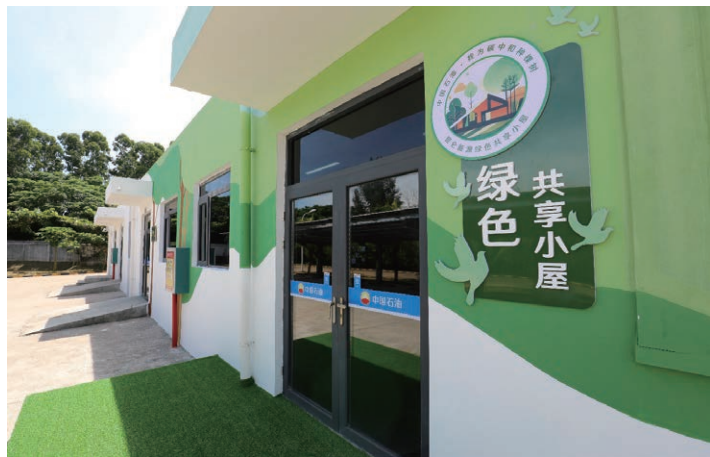
Kunlun Energy Hainan Green Shared Hut
