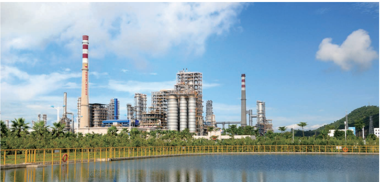
Guangxi Petrochemical 3.5 Mt/a catalytic cracking unit
