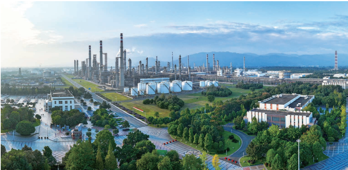
Sichuan Petrochemical plant area
