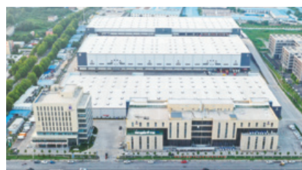
42 Zhengzhou Erqi Project
