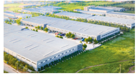
21 Tianjin Xiqing Project
