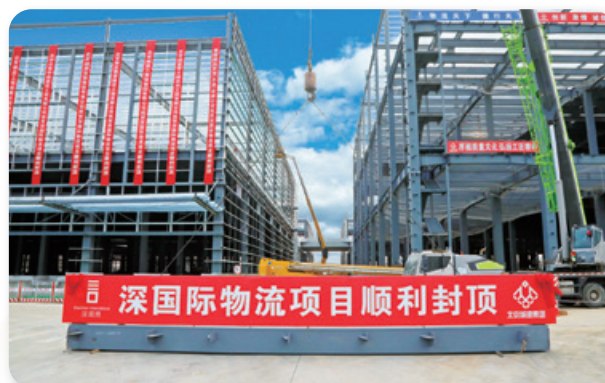
SZI Beijing Southwest Integrated Logistics Hub (Phase I) Intelligent Logistics Center
