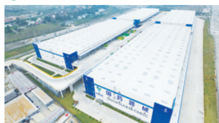
15 Foshan Gaoming Project
