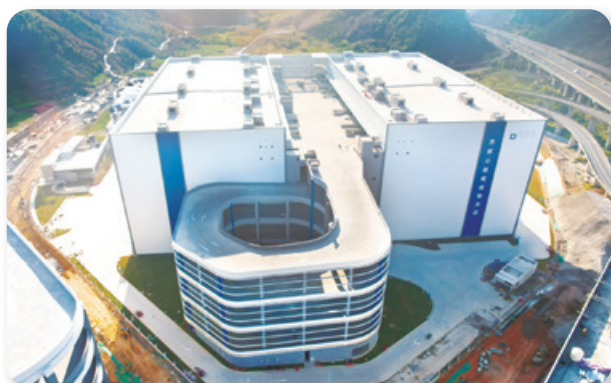
SZI Western Highway Freight Logistics Hub
