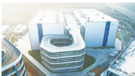
2 SZI Western Highway Freight Logistics Hub
