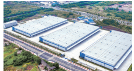
33 Chongqing Shuangfu Project
