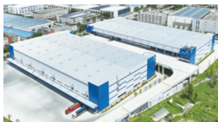
37 Chengdu Wenjiang Project
