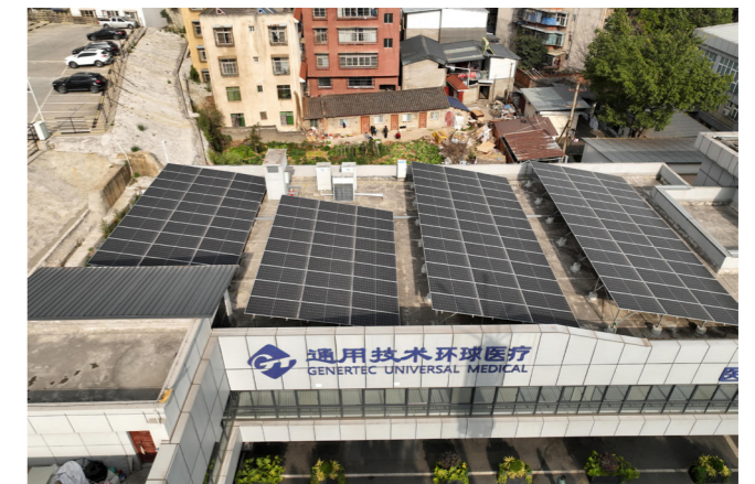
Xichang Hospital L-shaped medical technology building rooftop solar photovoltaic power generation system
