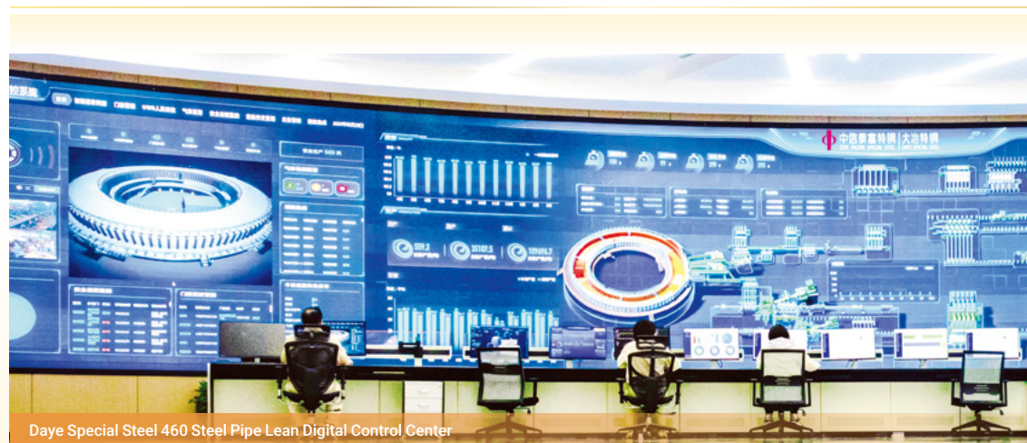
Daye Special Steel 460 Steel Pipe Lean Digital Control Center
