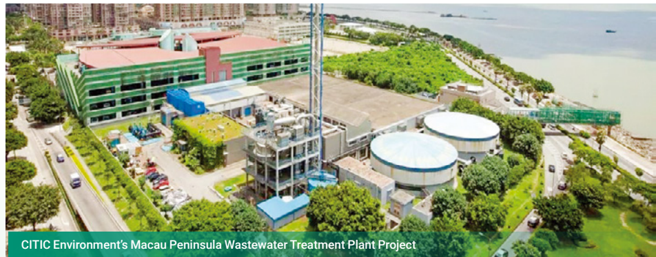
CITIC Environment's Macau Peninsula Wastewater Treatment Plant Project
