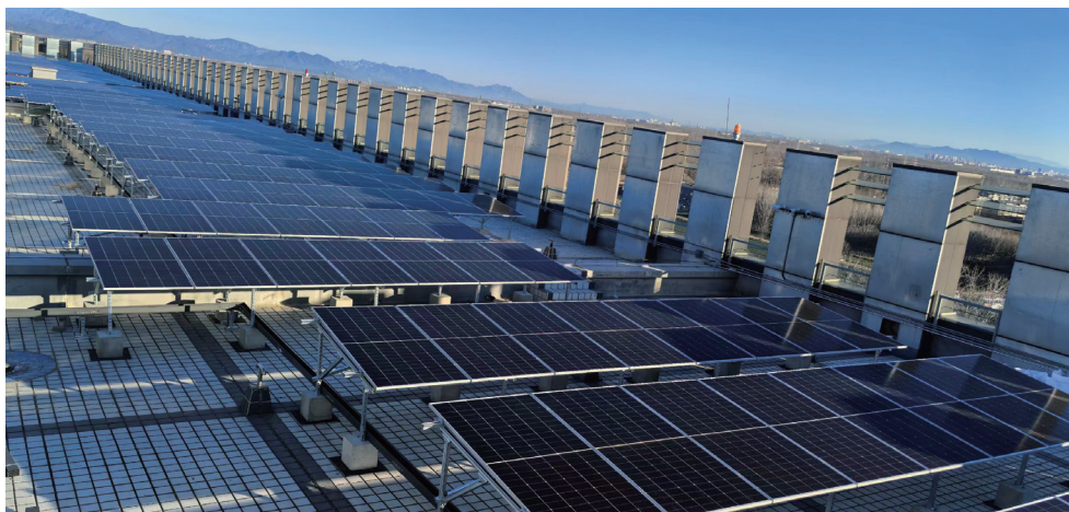
Rooftop solar photovoltaic construction in TravelSky High-Tech Industrial Park
