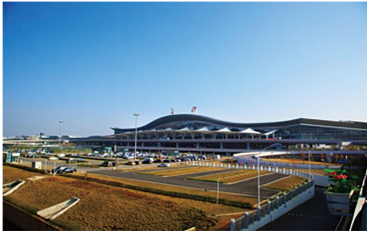
Distributed intelligent energy application technology and equipment
