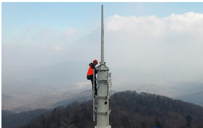
Base Station Construction for Harbin Asian Winter Games
