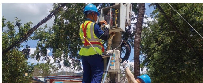
After the Typhoon, Engineers Are Racing Against Time to Repair Communication Stations
