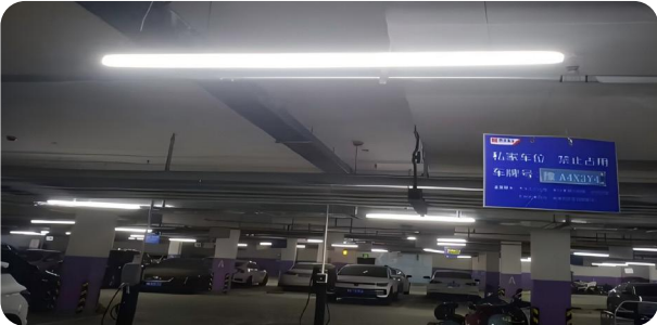
Basement Lighting System Upgraded with Energy-Efficient Fixtures
