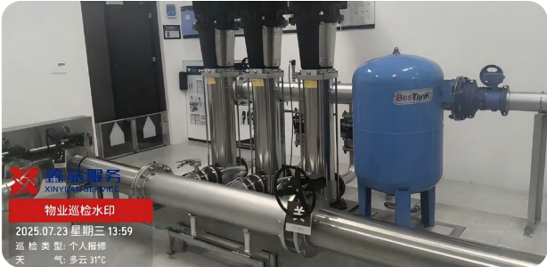
Water Pump Energy-Saving Optimization and Equipment Retrofit
