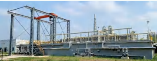
Wastewater Recycling Treatment Station of Guorui Pharmaceutical
