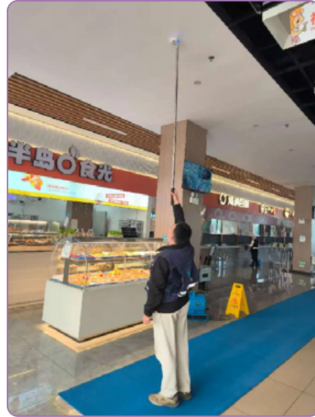
Inspection of fire safety system elements
