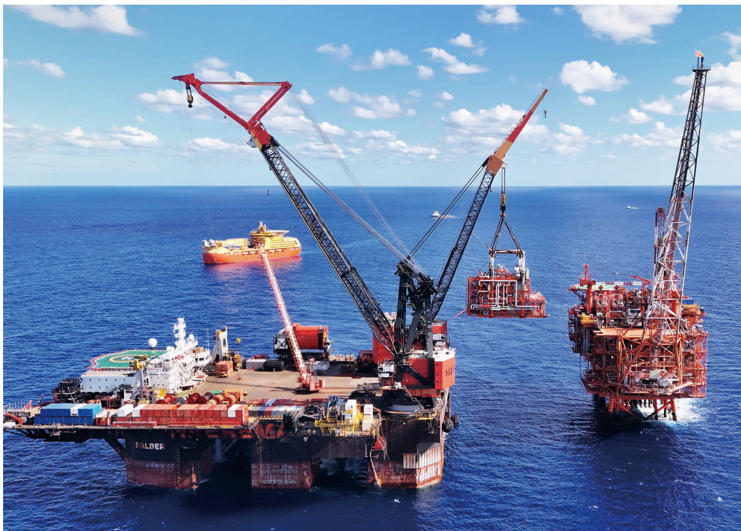
KLN Project under the Group's IFF division completed the one-stop offshore transportation and installation of a 1,700-ton gas compression module on the Sabratha Offshore Platform in Libyan waters in October 2025
