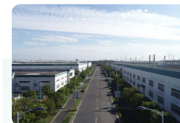
Taizhou, Jiangsu-Lead-carbon & Lead-acid Production Base
