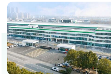
Xiangyang, Hubei-Lithium-ion Battery Production Base
