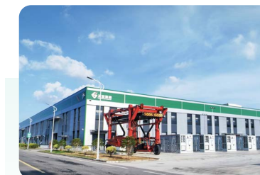
Taizhou, Jiangsu-Energy Storage System Integration Base--Domestic
