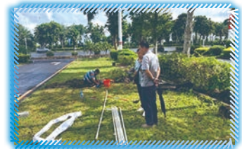
Renovation of reclaimed water pipes in green areas 綠化區域中水管道改造
