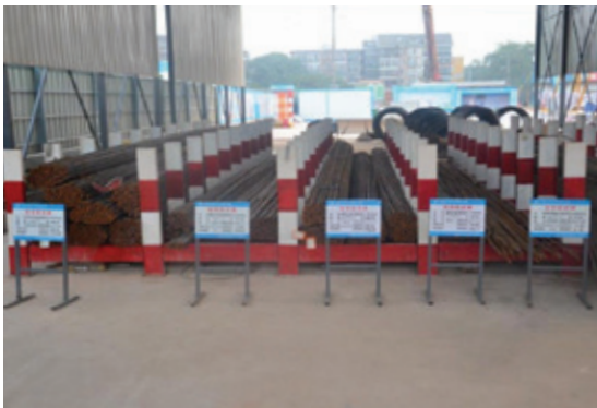
Rebar stacking rack
