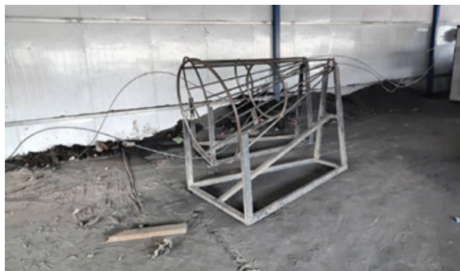
Protection for rebar straightening
