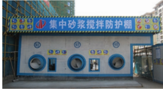
Setting up rain-proof and anti-smashing sheds
