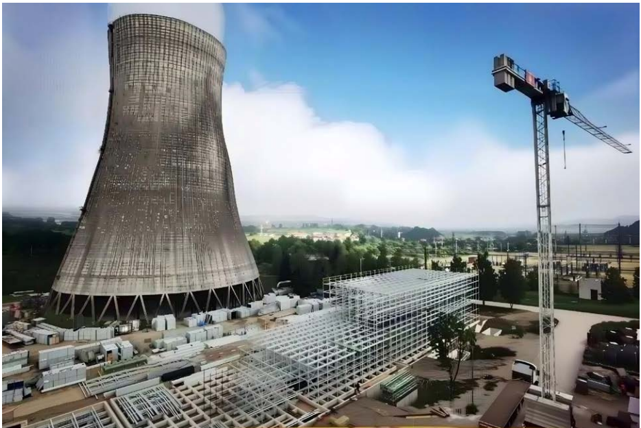
PICC undertook the environmental protection renovation project of Pljevlja Power Plant in Montenegro
