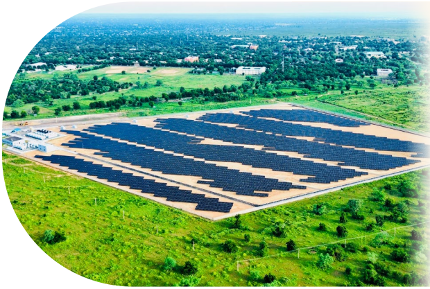
Nigeria's largest diesel-photovoltaic-storage integrated energy project was officially put into commercial operation. The completion and operation of this power station not only effectively alleviated the local power shortage but also injected strong impetus into the local sustainable development.
