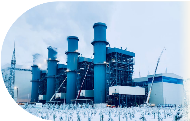
The Mingachevir Combined Cycle Project in Azerbaijan was officially put into operation, with DEC providing four F-class waste heat boilers and their auxiliary equipment for the project.
